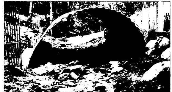
This open bottom culvert allows stream flow and aquatic organism passage (note people working by huge culvert).
